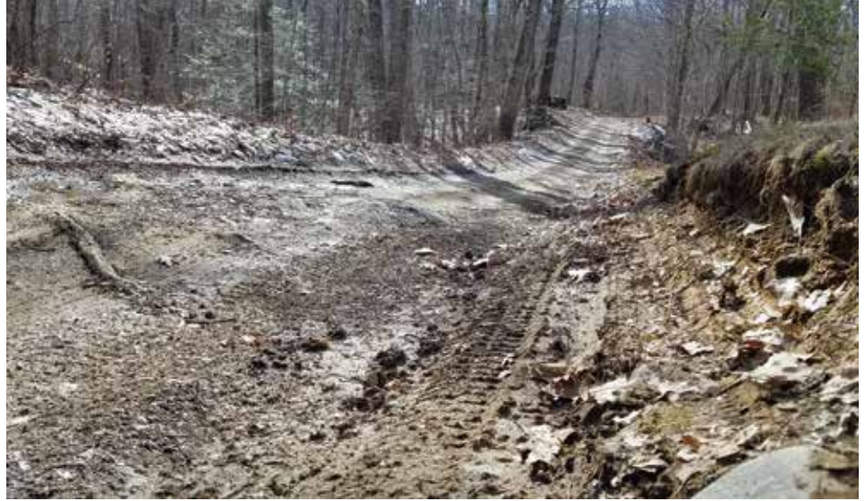
Erosion can creep up on you. This driveway used to be level with the ground to the right of the photo.
